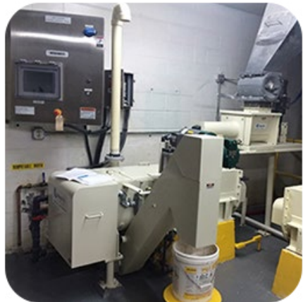
Nebraska City WWTP, NE
