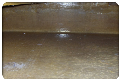
Sump after Acid Wash
