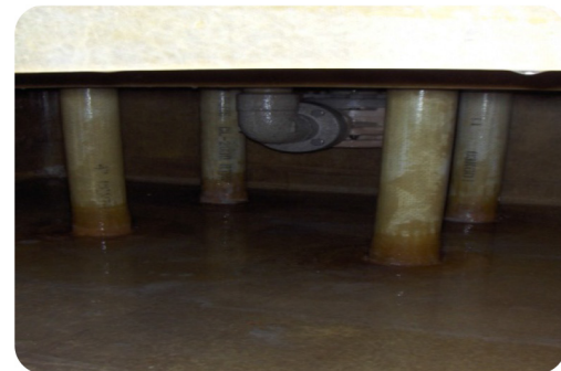
Sump After Acid Wash
