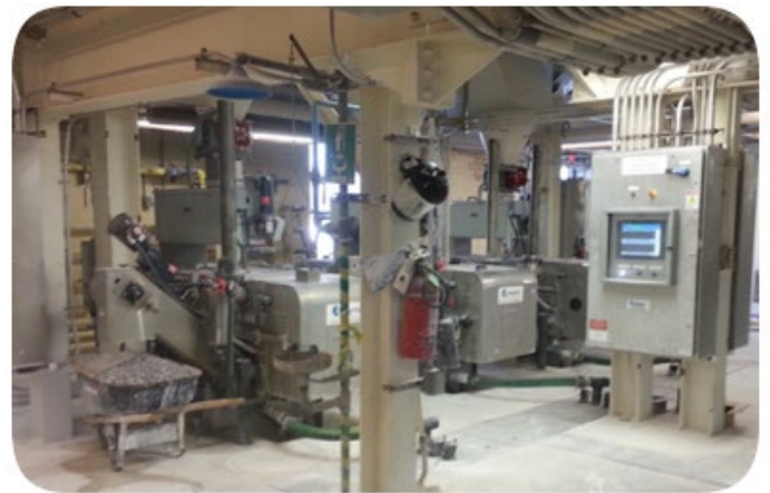
After the new paste-type lime slaker systems were installed, operators can start and stop each system without leaving the control room. Operators and other plant personnel can monitor many aspects of each slaker system from their desk computer. A detailed alarm is reported to the system controls and is displayed on the local screen, complete with history.
