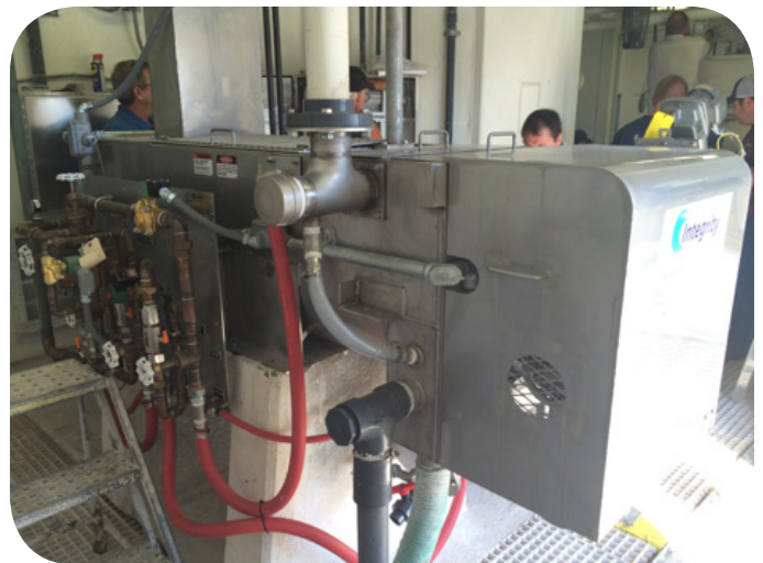
Patent-pending, pre-assembled water panel
