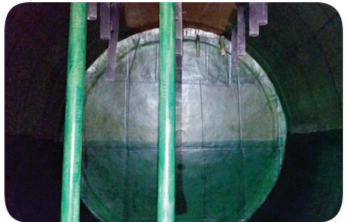
Storage tank interior after repairs and relining
