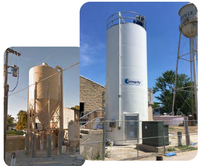
*Woodville upgraded their aging hydrated lime container, shown left, with a new IMS silo featuring integrated level detectors and seamless connectivity with their chemical feed system.*
