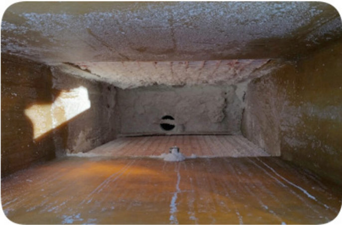
Temecula Valley Scrubber Interior Before/After Acid Wash
